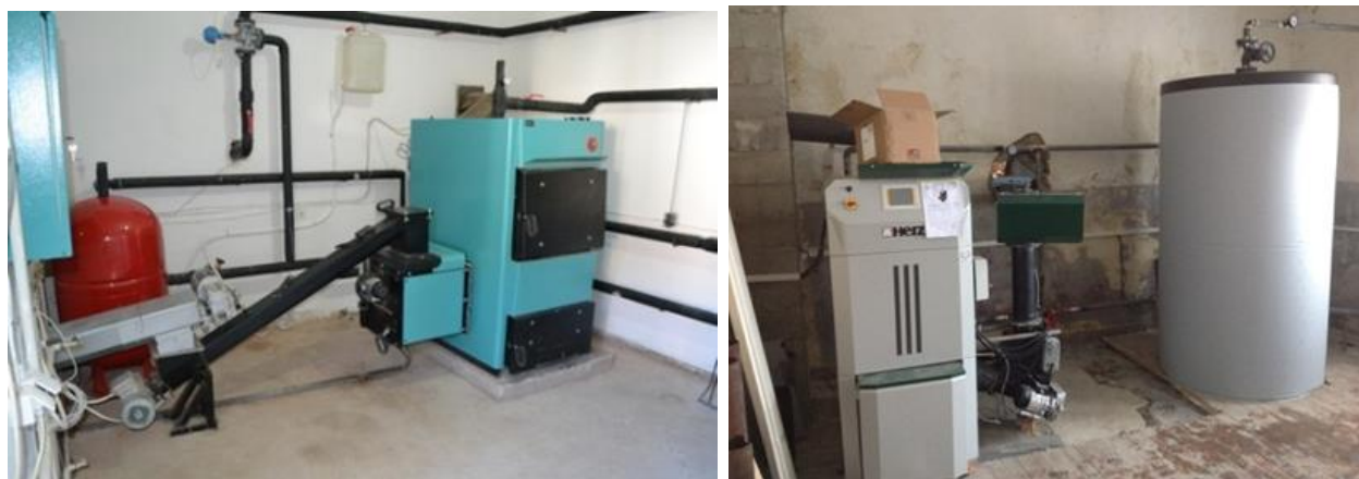
Figure 30: Woodchips based boilers for the central heating systems installed for the schools
